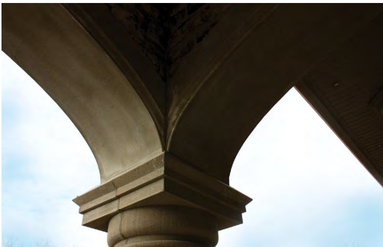
Private Residence, Conestogo Contractor: Van-Del Contracting Ltd.
