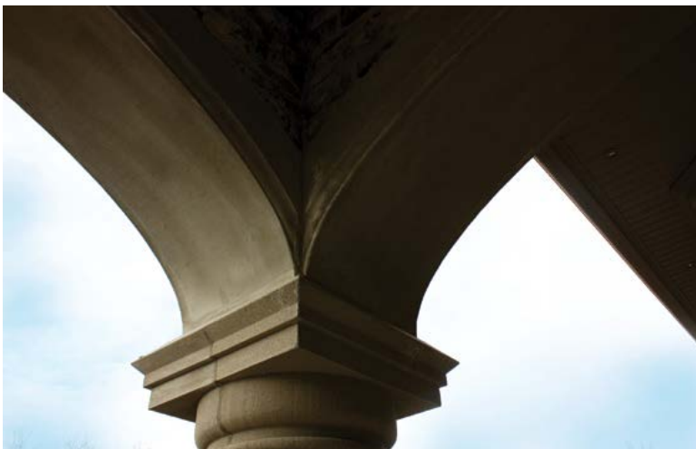
Private Residence, Conestogo Contractor: Van-Del Contracting Ltd.
